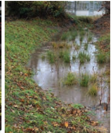
Vegetated Swale University of Victoria
