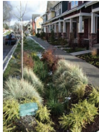
Street side Vegetated Swale High Street, Seattle
